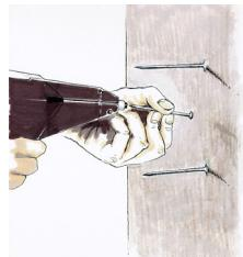
Insert the SP2-TC pin in the magnetised tip of the pinwelder PW-33.
